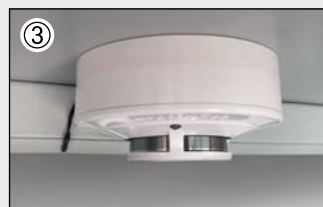
Smoke detector and temperature sensor
