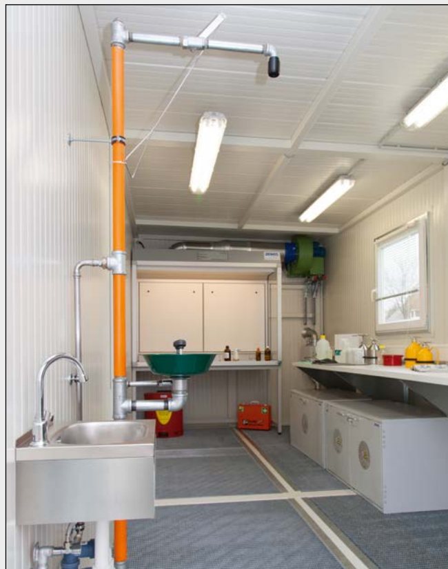
Sampling room with ventilation technology workplace and emergency shower. Additional safety is provided by fire-rated underbench cabinets for retained samples.
