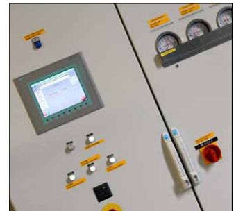
Main control panel with Siemens S7-300 PLC and 10" HMI screen
