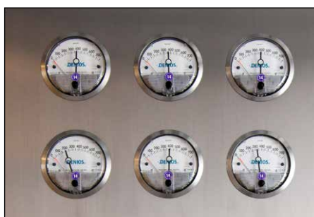
Monitoring of differential pressures, air speed and air quality, analogue or digital
