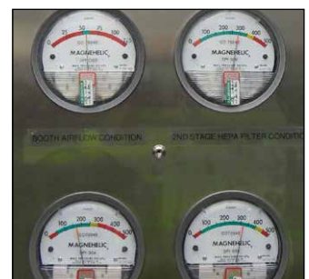
Magnehelic differential pressure gauge with marked areas for safe operation
