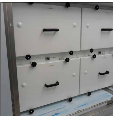
Filter housing for contamination-free filter replacement
