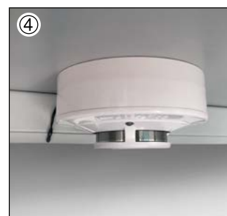
Temperature sensor sits directly behind the smoke detector
